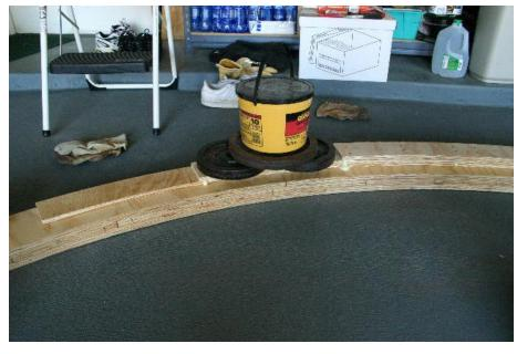
Since the dome ring used <sup>3</sup>/<sub>4</sub> inch plywood, I used 1-1/4 inch decking screws to secure each layer to the layer below. I glued and screwed each arc one at a time, working my way around the ring. I paired 2 screws (one near the outside radius of the arc, the other near the inside radius) at an approximate 8-inch
